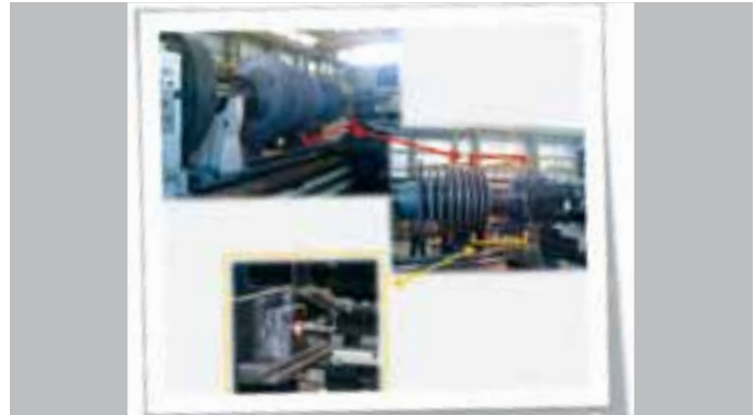
Removal of a core sample and repair of the removal site by a Friction Taper Hydro Pillar Processing platform developed specifically for this application at eNtsa. The cylindrical core sample removed from the turbine rotor disk allowed Eskom's engineers to accurately determine subsurface creep damage.
